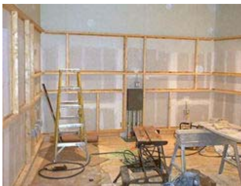
May: Master Control Room studio framing.
