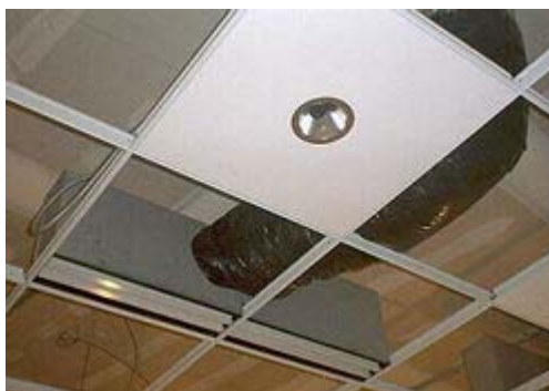
APRIL: New studio ceiling grid.
