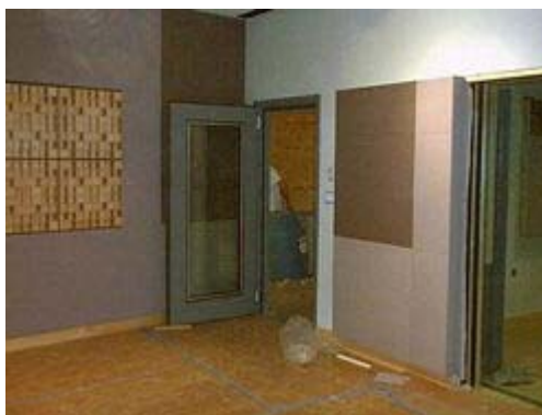
June: New Master control with temporary floor.
