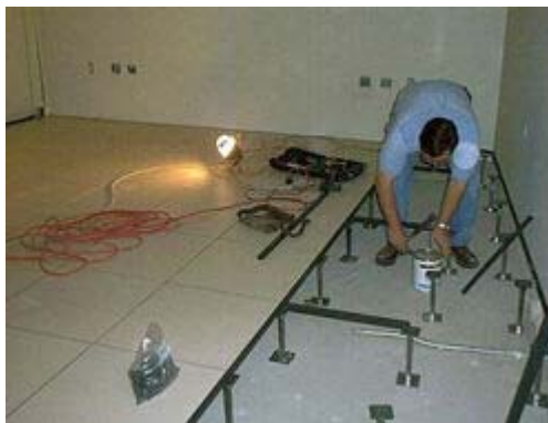
APRIL: New Engineering room floor.
